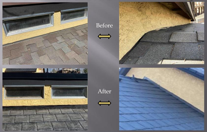
All About Stucco had to coordinate with roofers before and after install to cutback the stucco and then reskim it.
