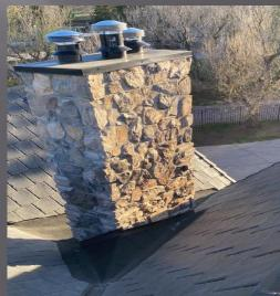
Woodward Masonry had to coordinate with roofers before and after install to cutback the stone to be properly install the chimney flashings
